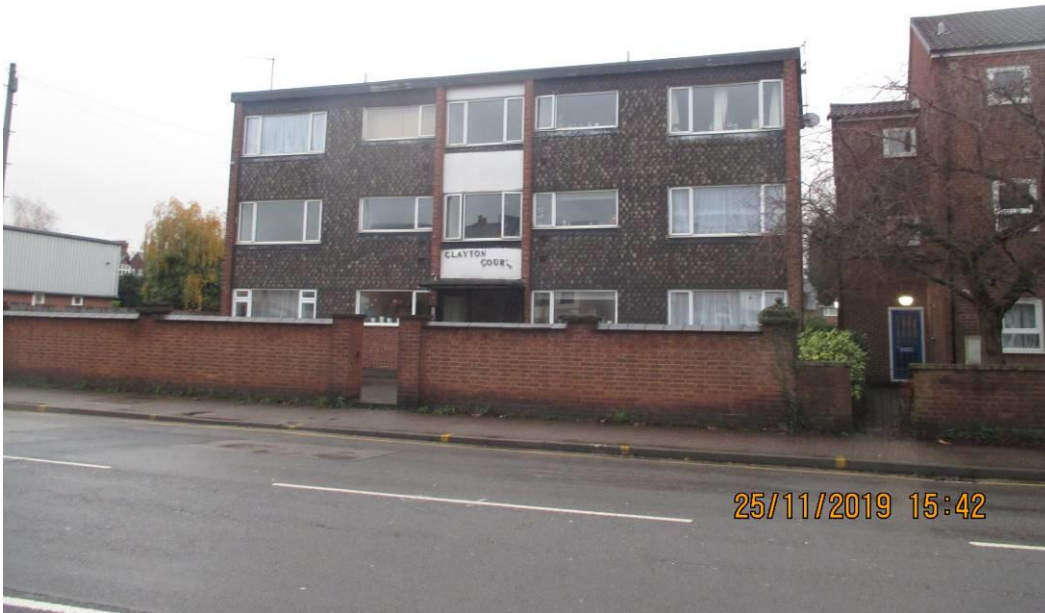
North west (front) of Clayton Court flats (wall to be removed)
