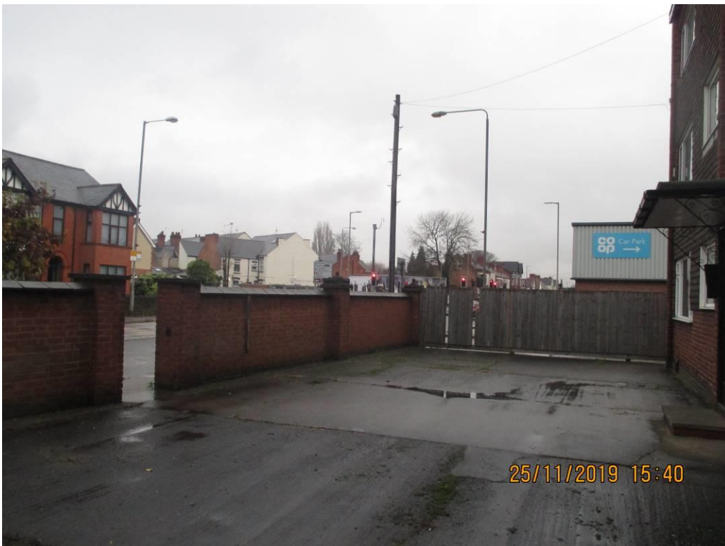
Facing north east of existing frontage (view of Co-op, Clayton Court flats to the right)
