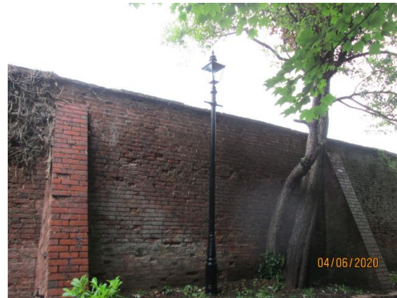
Lamp post and west boundary of the site.
