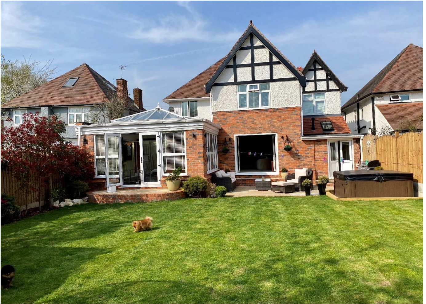
South (rear) elevation showing cattery removed
