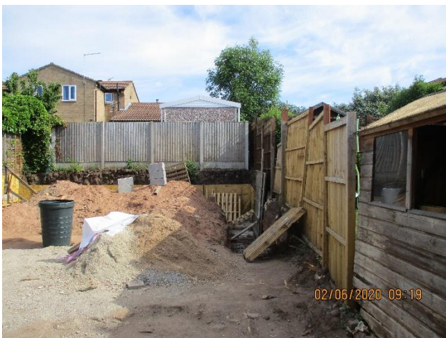
Rear and boundary with no. 8
