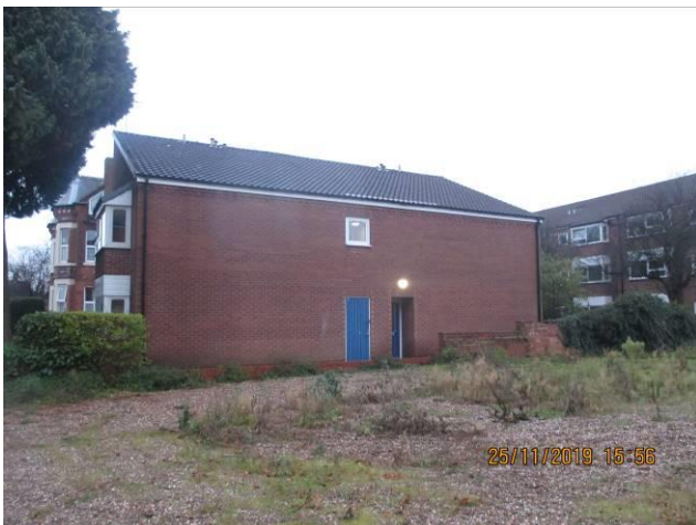
North east (side) elevation of Sovereign Court flats
