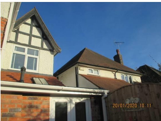
South (rear) elevation of main house and no. 233 to the right
