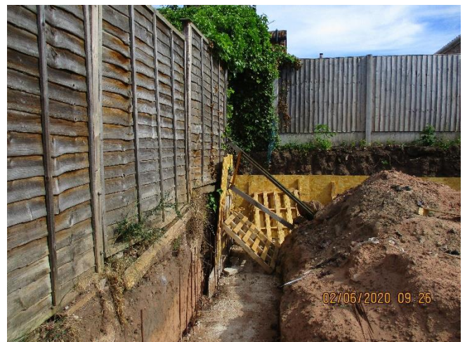
Rear garden works.
