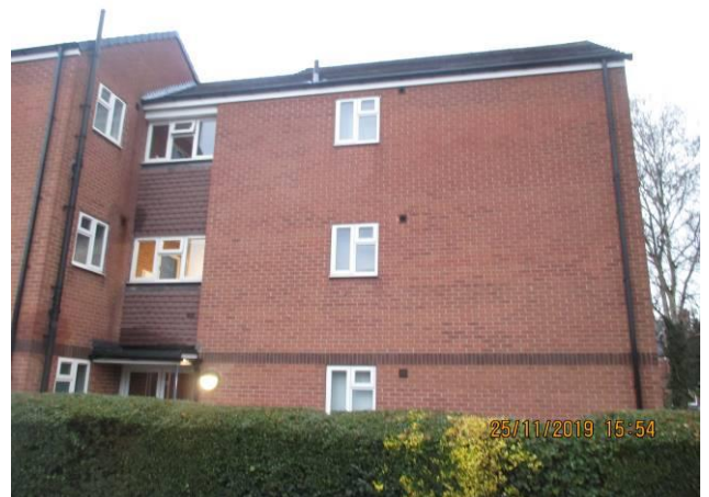
South west (side) elevation of Runnymede Court flats
