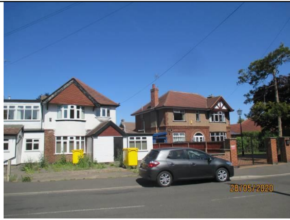
Relationship between site and 173 Attenborough Lane. Note the bins to the frontage which served the former care home
