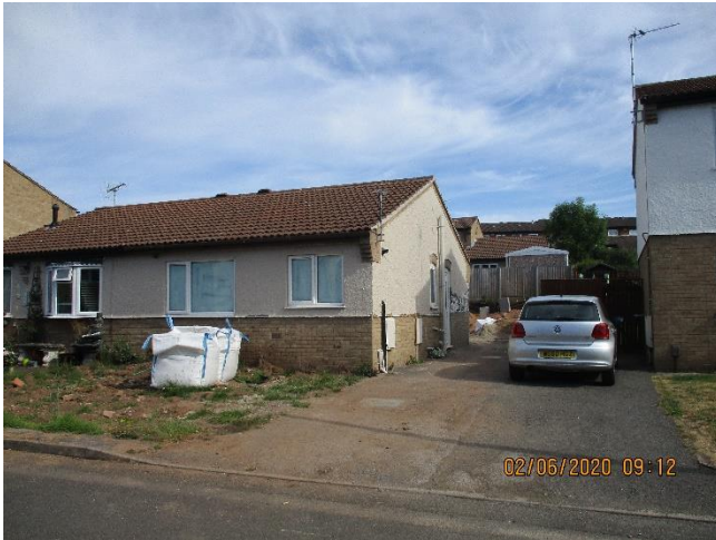
Front (south) and side (east) elevations.
