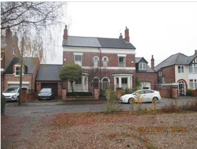
Facing south east (nos. 5 and 7 Grove Street)
